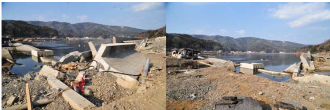
Fig. 2.2 Destroyed port facilities and general alteration of the shoreline in Mizuhama town (Lekkas et al., 2011)
